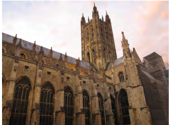
Bell Harry Tower, Canterbury. (Christopher John)
