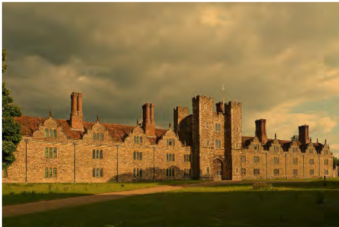
Knole House, Morton's principal residence in Kent. (John Wilder).
