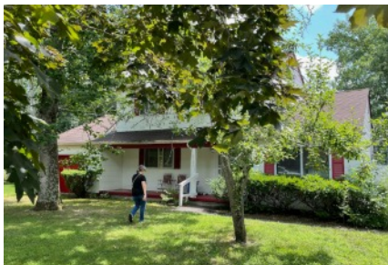
View of Cape Cod from street.
