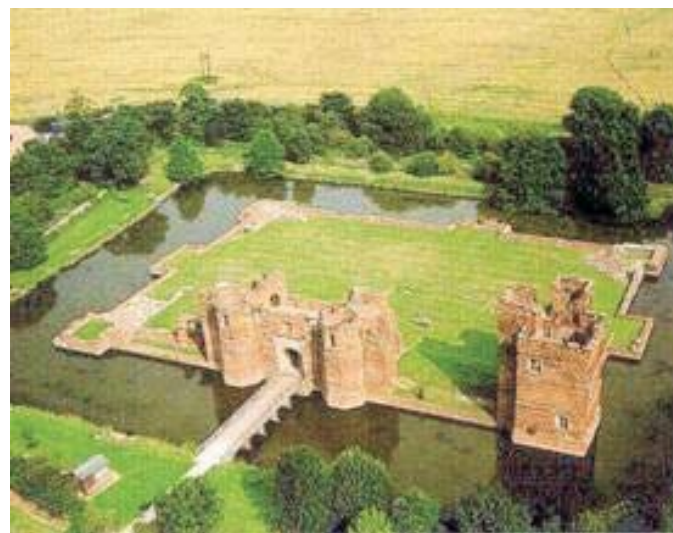
Figure 11: Twin aerial views of the Castle. In the picture on the right, the remains of the original curtain wall can be seen between the gatehouse and the tower. As is evident, these connecting walls did not rise directly from the moat but were set back leaving a rampart which would have been protected by a lower wall.
