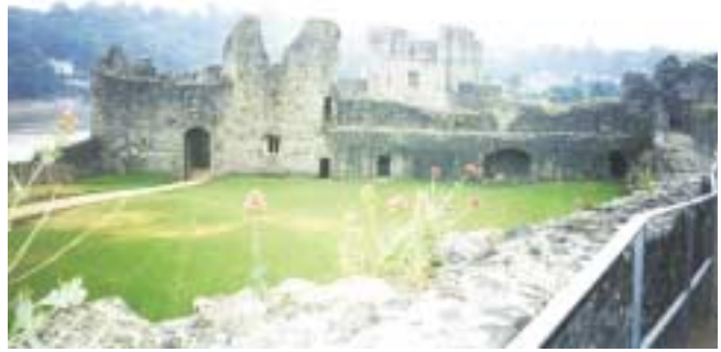
Chepstow Castle: A view from the curtain wall across the middle bailey and the gatehouse
